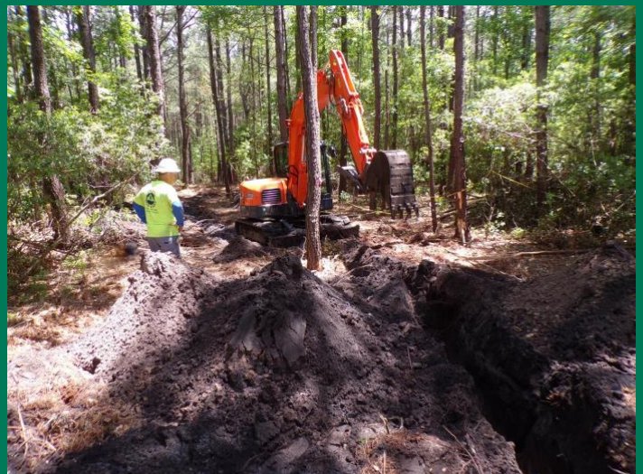
In June 2019, during soil sampling in the northern area of the Site, a Multistate Trust contractor's team (left) collects soil samples using a Geoprobe drilling rig. In May 2018, a Multistate Trust contractor's team (right) installs trenches to collect soil samples needed to evaluate subsurface conditions.
