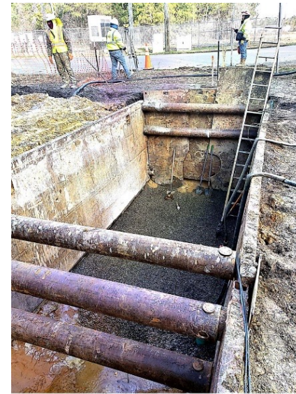
Brunswick County contractor installing Wastewater Treatment Plant Force Main
